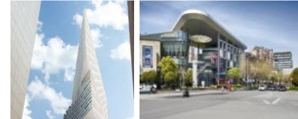
Quay Quarter Tower | Jinqiao Life Hub, Shanghai
